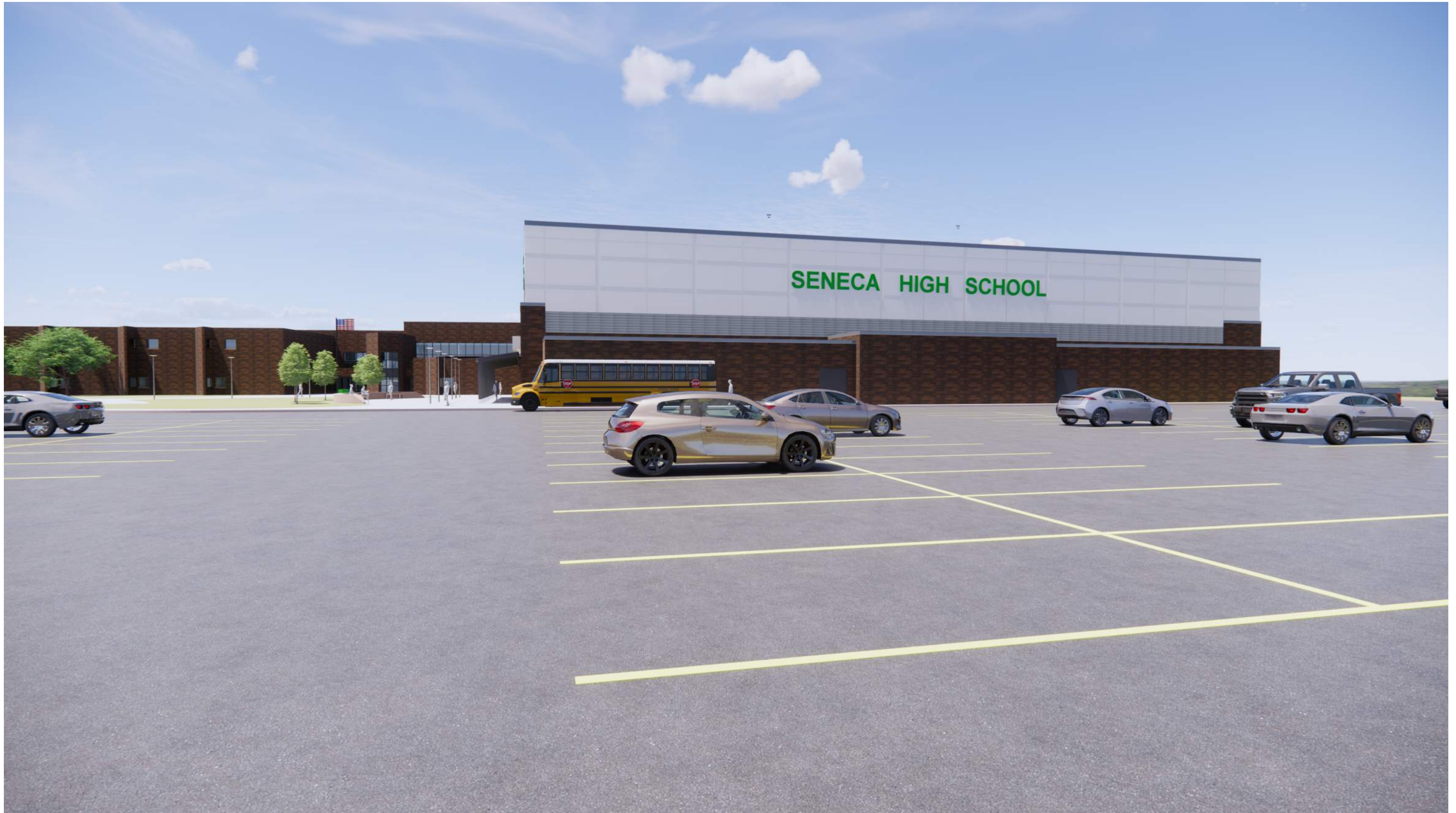
East Exterior View
